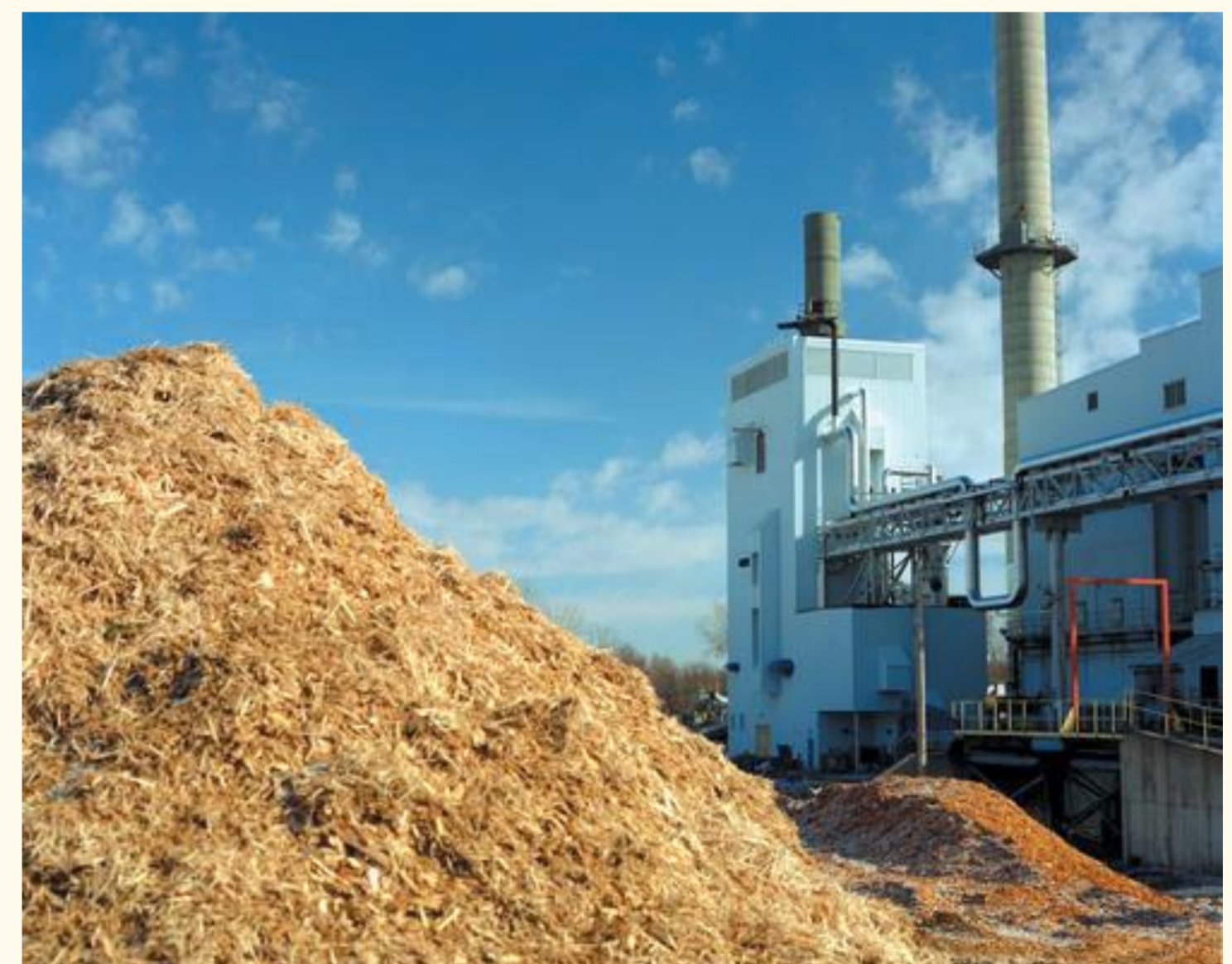
Fig. 1. Biomass power plant
